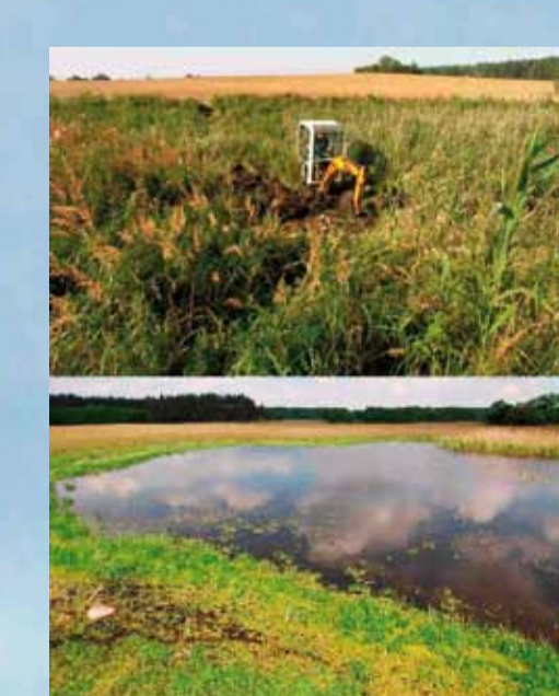
Drained wetland before and after the removal of artificial drainage. Foto: Rüdiger Mauersberger
