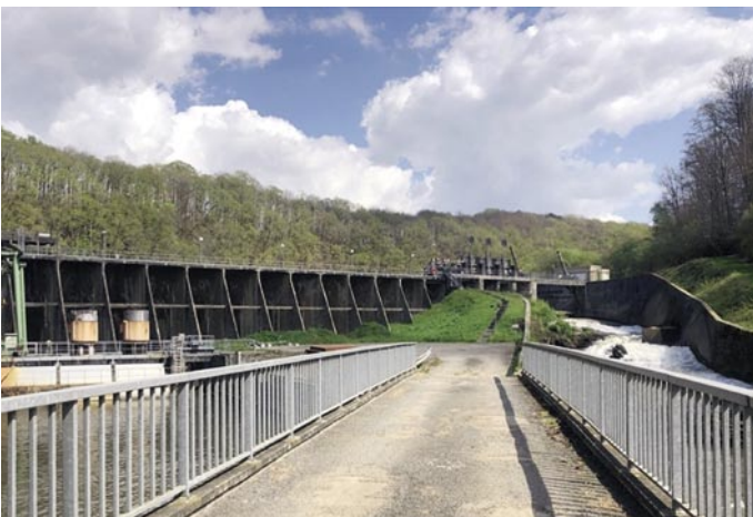
La Roche-qui-Boît dam (EDF Property), with an opening on the right side and the factory on the left side.
