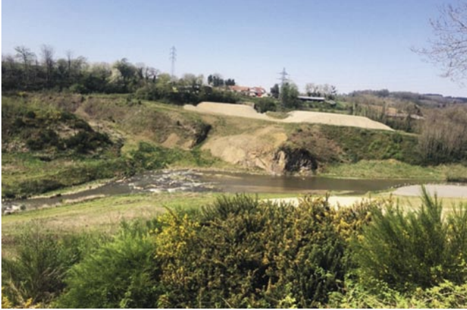
Former site of the Vezin's dam, downstream the reservoir, demolished in 2021.
