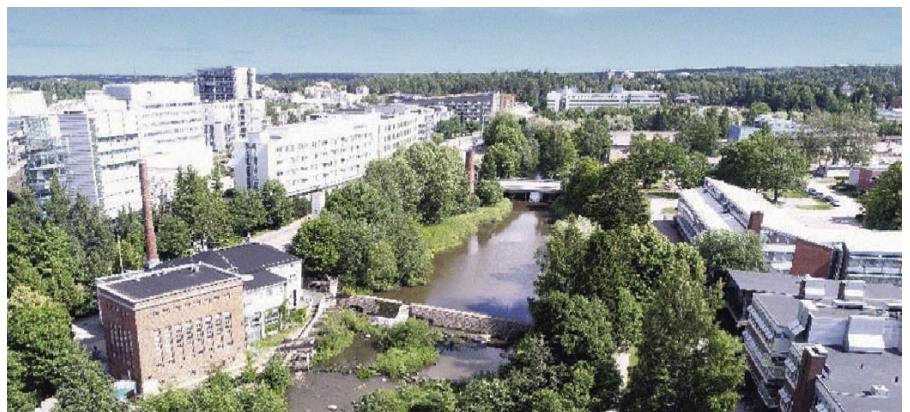
An aerial photograph taken from southwest. In the centre is the dam and next to it on the left side is Vernissa. (The removal of a culture-historical Tikkurila dam for improved resilience of urban nature, Tiia Valtonen, 2017)
