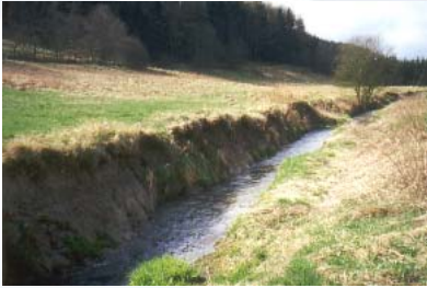
(1) 1997: The Ruwer downstream of Kell am See – deepened and straightened
