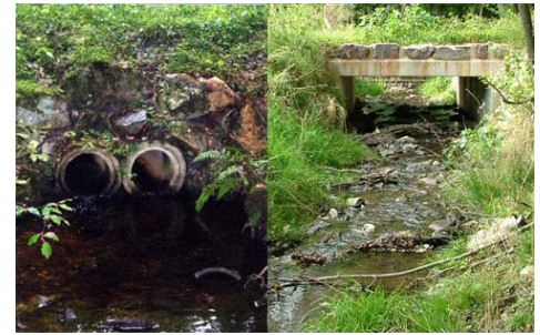
(4) Pipe passage at the Weierbach is made „permeable“
