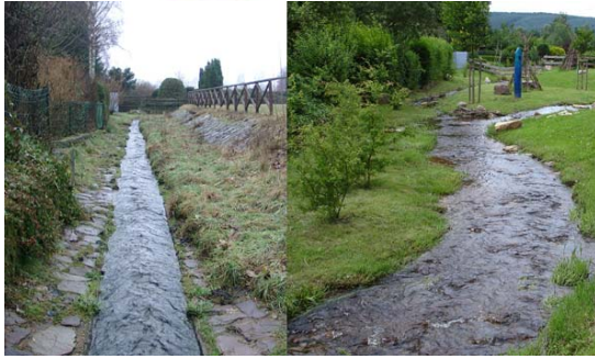
(3) The Eselsbach, tributary of the Ruwer, before and after restoration
