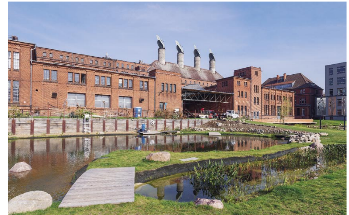
Green roofs and artificial water surfaces on the grounds of IGG Malzfabrik in Schöneberg ensure the retention of rainwater as well as its usage as process water.
