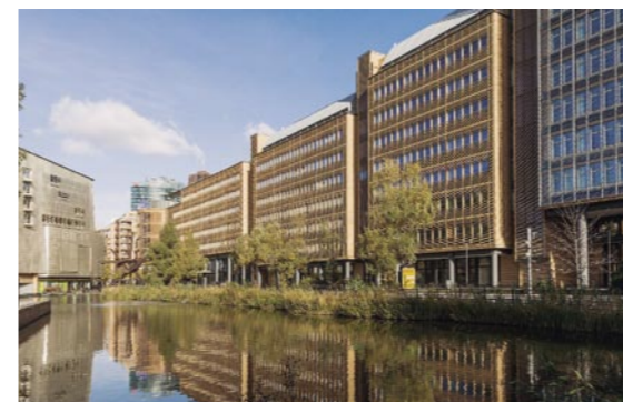
To prevent excessive spillover into the Landwehr Canal, the overall ecological concept at Potsdamer Platz merges green roofs and ponds, as well as rainwater storage tanks for rainwater use as process water.
