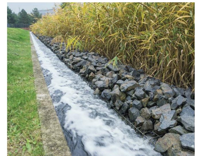
The soil filter with a rainwater purification basin in Adlershof minimises pollution discharge into the Teltow Canal by introducing the purified rainwater into the water body with a time delay.
