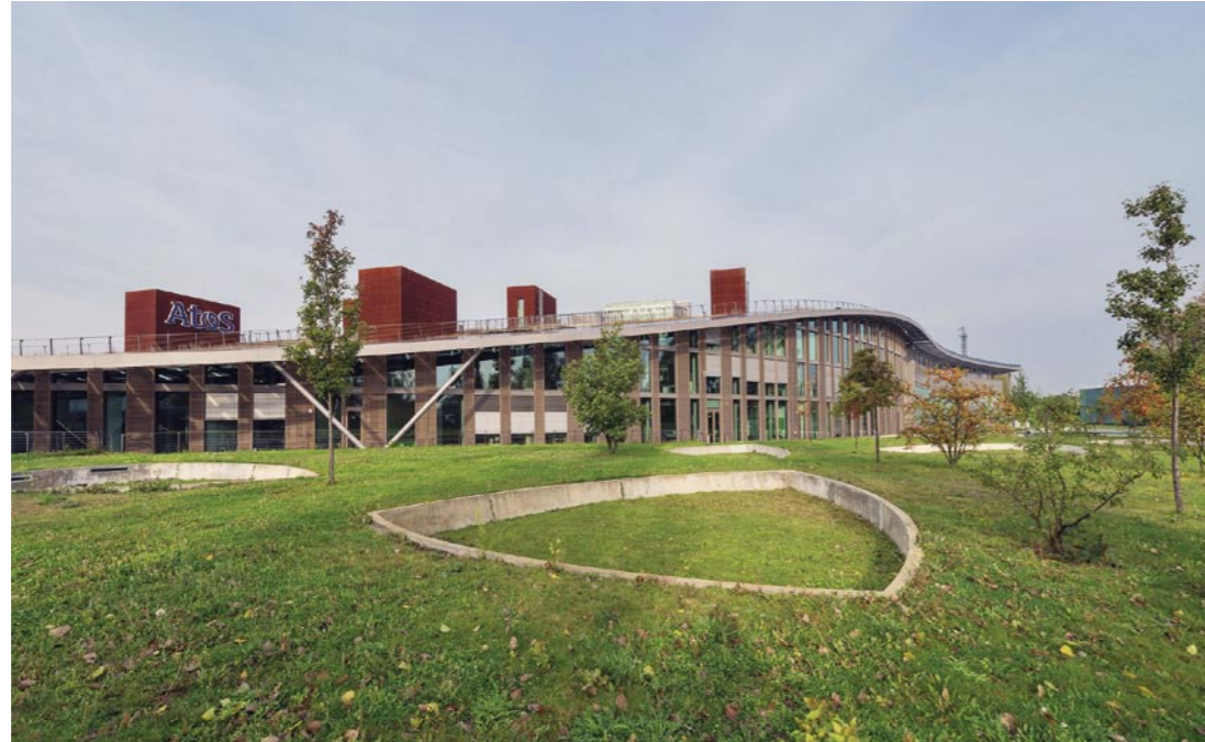
The former Solon site in Adlershof – green roofs, ponds and infiltration ditches keep the rainwater on the property entirely.
