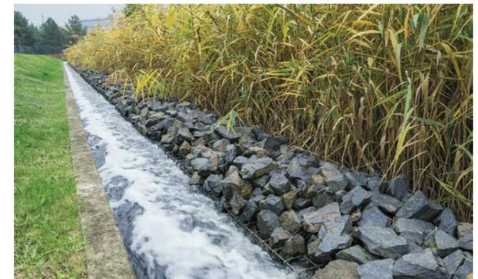
The soil filter with a rainwater purification basin in Adlershof minimises pollution discharge into the Teltow Canal by introducing the purified rainwater into the water body with a time delay.
